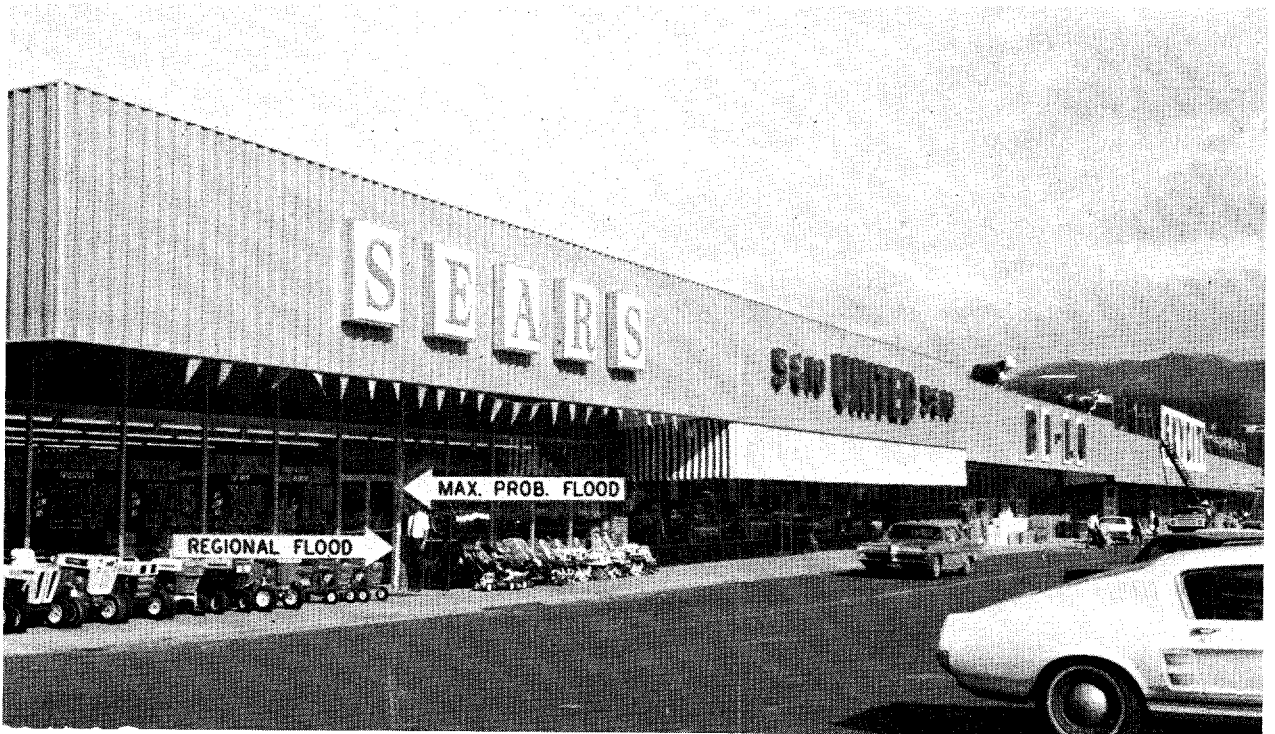
Figure 9. --FLOOD HEIGHTS AT RICHLAND CREEK SHOPPING CENTER
