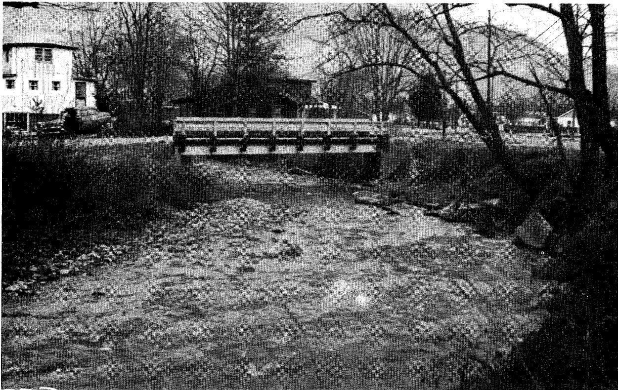
Figure 7.--ALLEN CREEK BRIDGES IN SOUTHERN WAYNESVILLE
