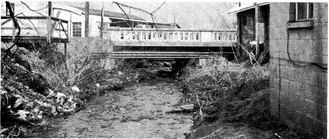
Figure 4. --CAMP BRANCH BRIDGES
