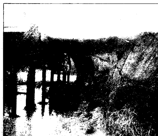
1940 Flood damage to N.C. Highway 18 bridge on Hunting Creek.
