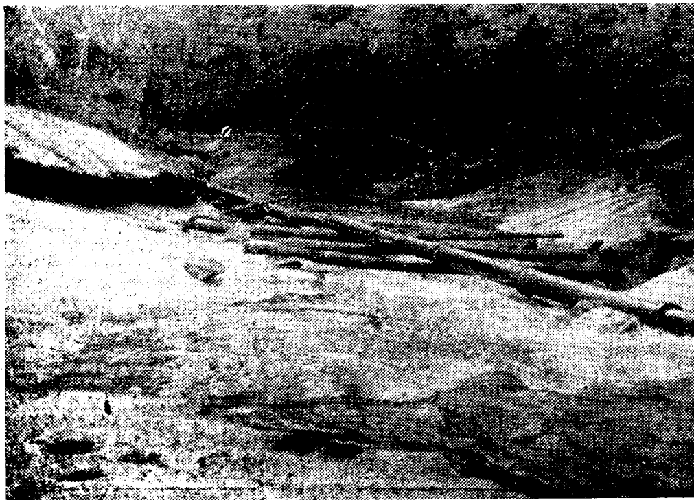
1940 FLOOD DAMAGE TO MORGANTON'S MAIN WATER LINE
