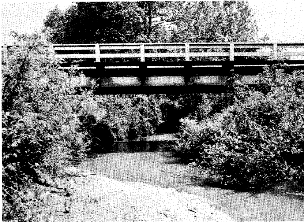
New Laurel Road Bridge
