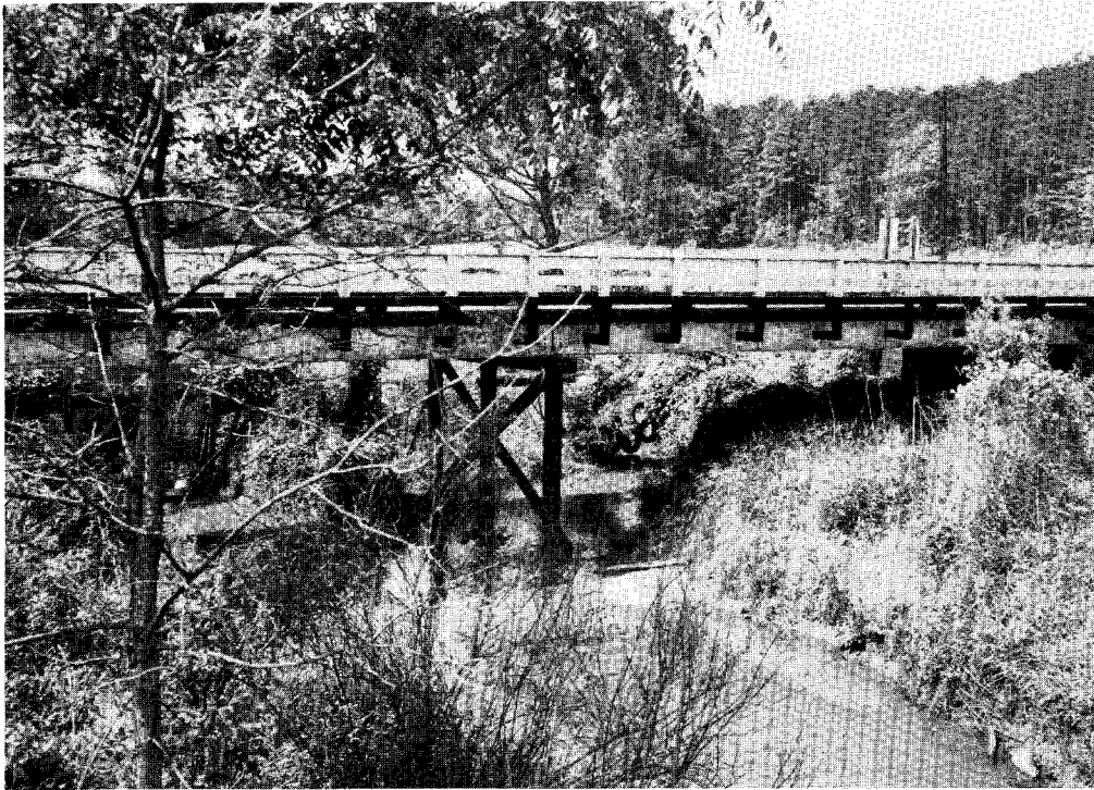
Bethel Street Bridge
