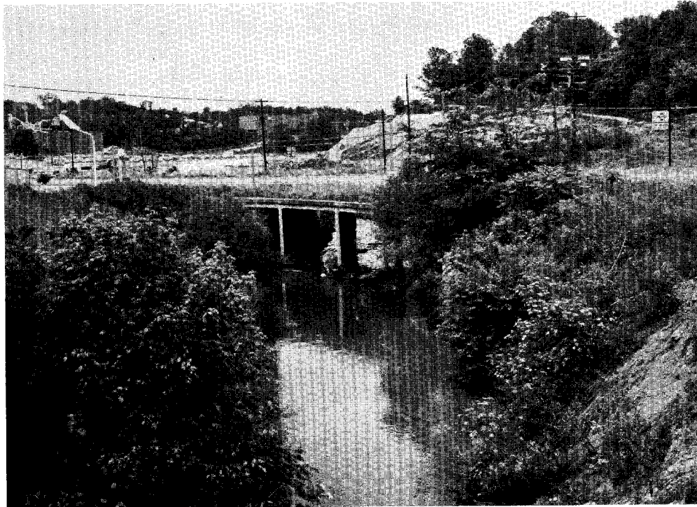
N. C. Hwy. 18 & Sterling Street Culvert
