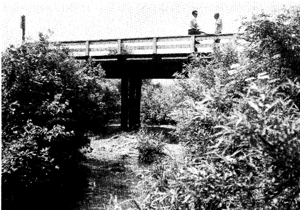
Bethel Road Bridge
