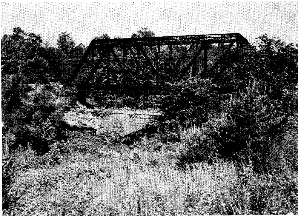
Natural obstructions which increase flood heights.
