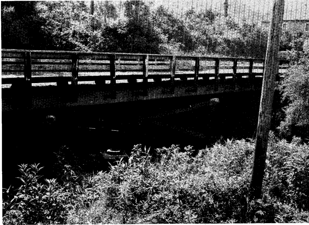
Bethel Road Bridge
