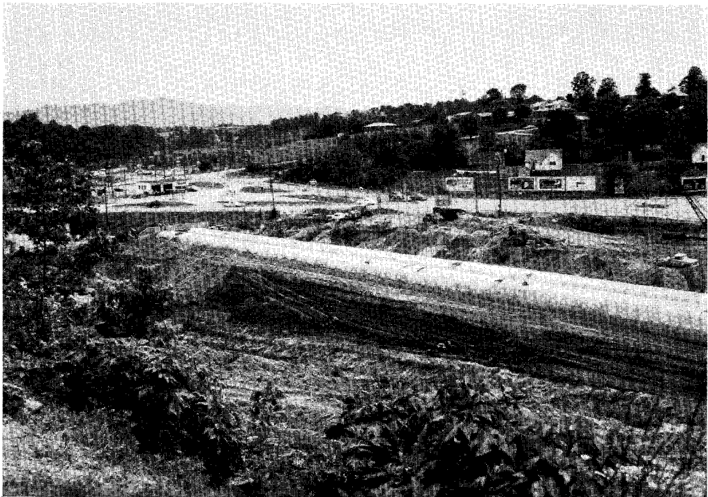
Figure 2 FILL IN THE FLOOD PLAIN Fill in the flood plain reduces the natural flow area and may increase future flood heights.
