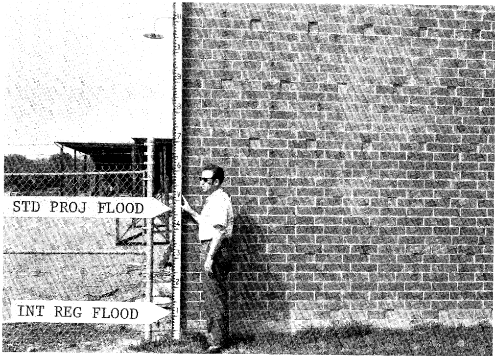
Arrows show approximate heights that would be reached by the Standard Project and Intermediate Regional Floods at an industrial building upstream from Bethel Road.
