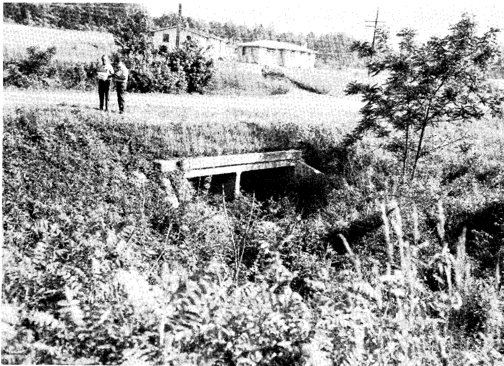
U. S. Hwy. 64 & 70 Byp. & Fleming Drive Culvert
