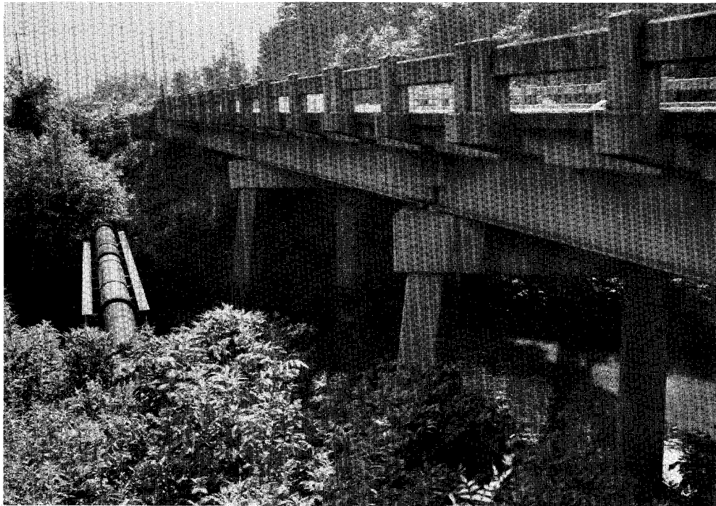
Fleming Drive & U. S. Hwy. 64 & 70 Byp. Bridge
