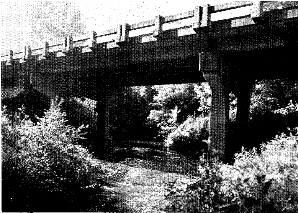
East Union Street & U. S. Hwy. 64 & 70 Bridge
