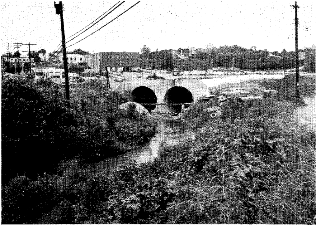
Figure 1 FLOOD PLAIN ENCROACHMENT Obstruction to flow increases future flood heights.
