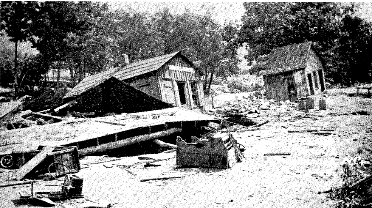
Figure 7. --BUILDINGS DEMOLISHED AT SWANNANOVA, JULY 1916
