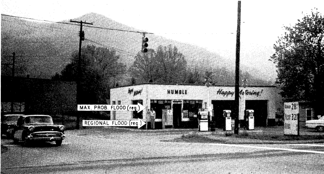
Figure 13. --FLOOD HEIGHTS AT WHITSON AVENUE
