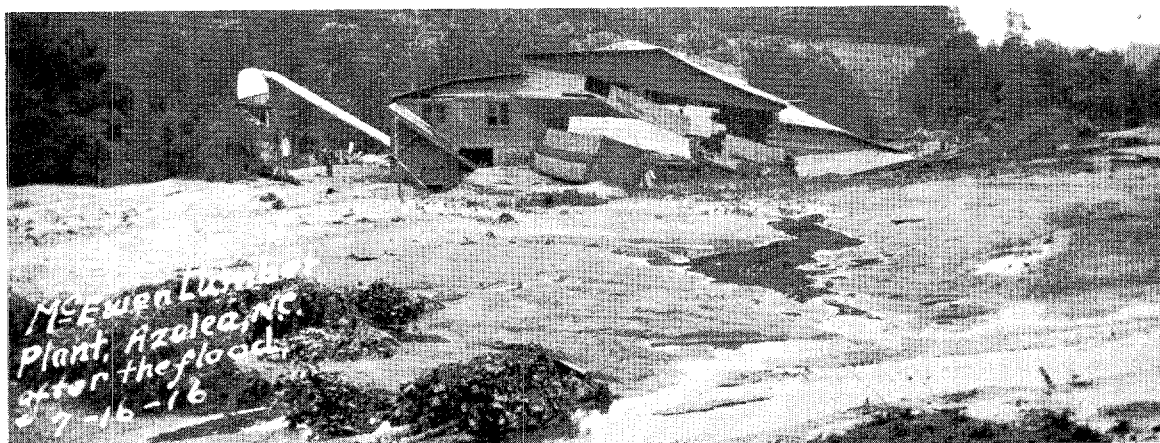
Figure 4. --WRECKAGE OF LUMBER PLANT, JULY 1916
