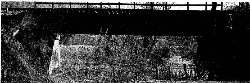
Southern Railway bridge at Mile 21.33, upstream side.
