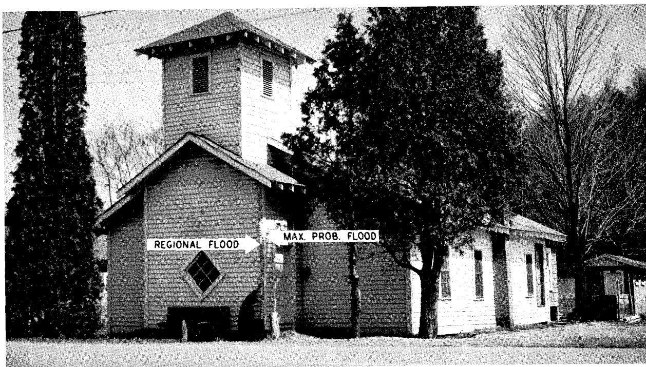
Figure 13. --FLOOD HEIGHTS ALONG BLACK MOUNTAIN AVENUE
