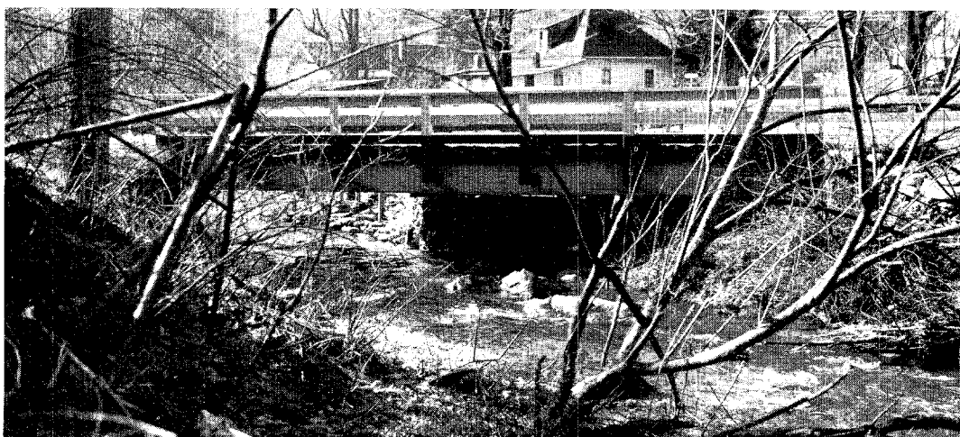
Flat Creek Road bridge at Mile 1.38, upstream side.
