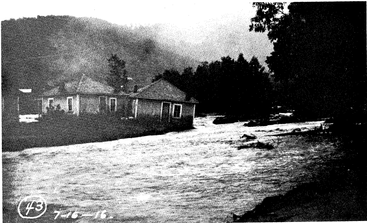
Figure 7. --FLOOD EFFECTS ON FLAT CREEK, JULY 1916
