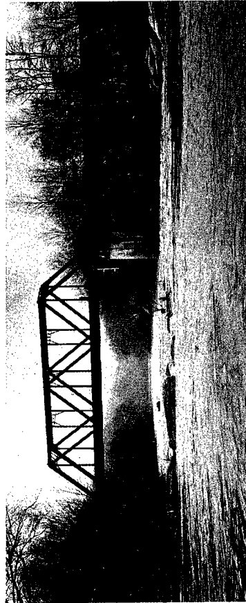
(a) Upstream side of bridge across Tuckasegee River near crest of flood of August 30, 1940. The crest level was about a foot above the underclearance.
