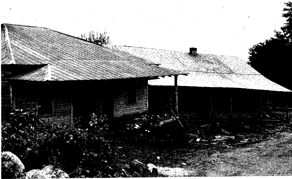
Figure 8. --BRYSON CITY BUILDINGS AND HOMES WERE FLOODED IN 1940
