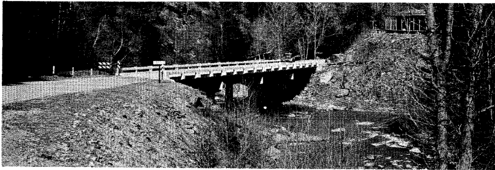
State Highway 209 bridge across Spring Creek
