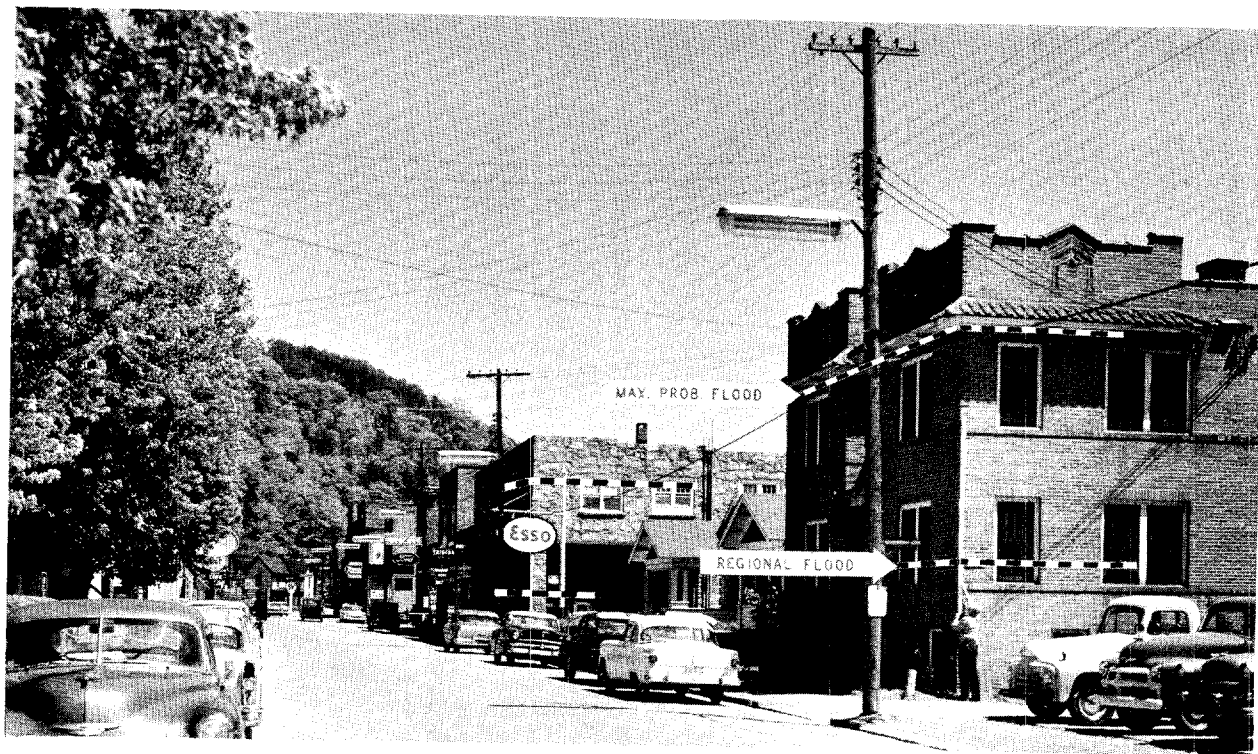
Figure 14. --FLOOD HEIGHTS ALONG MAIN STREET
