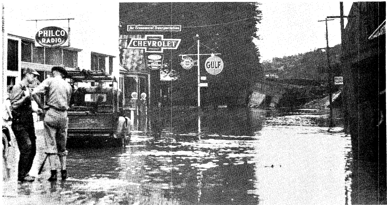
Figure 6. --BUILDING DAMAGE IN 1940 FLOOD
