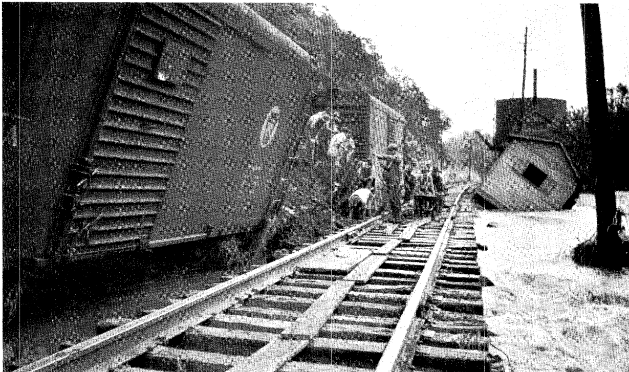
Figure 11. --RAILROAD TRACK DAMAGE IN 1940
