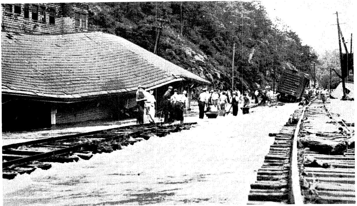
Figure 10. --SOUTHERN RAILWAY DAMAGE IN 1940
