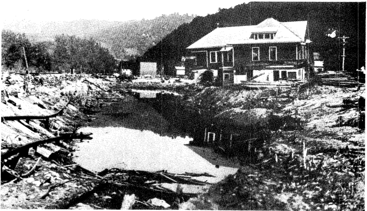
Figure 4. --DESTRUCTION BY 1916 FLOOD AT MARSHALL
