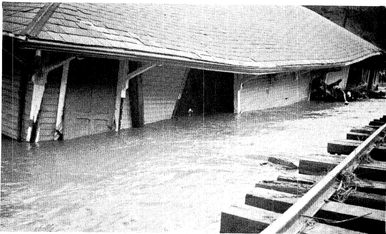
Figure 9. --SOUTHERN RAILWAY DEPOT AFTER 1940 FLOOD
