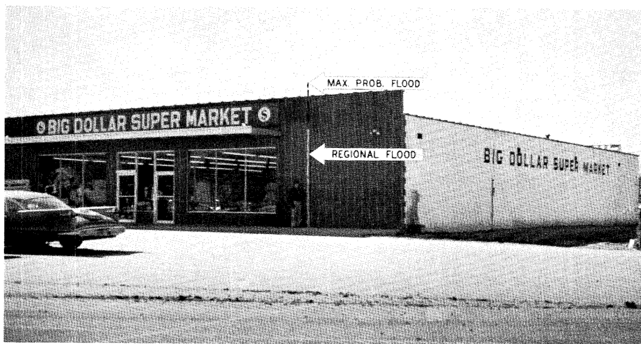
Figure 12. --SUPER MARKET ON RIGHT BANK OF LITTLE TENNESSEE
