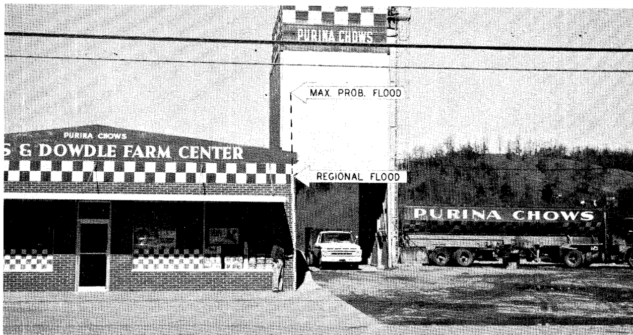
Figure 13. --FARM CENTER BUILDING ON U. S. HIGHWAY 23, 64, 441
