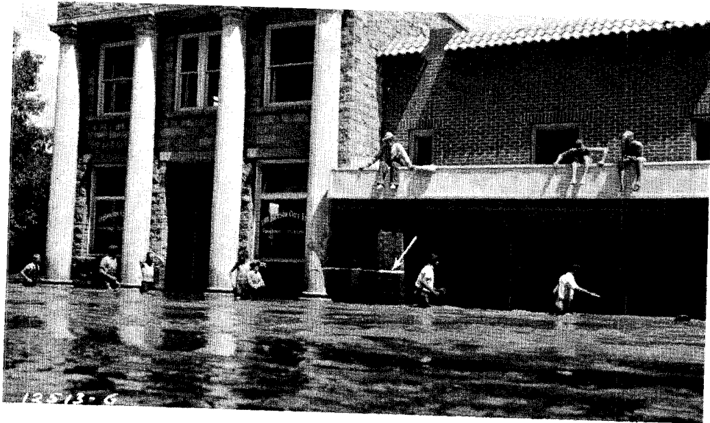
Figure 2. --BRYSON CITY BUSINESS BUILDINGS FLOODED
