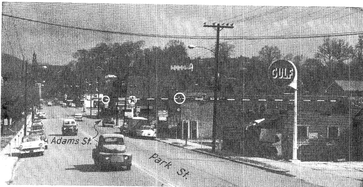
Figure 6.--PARK STREET, CANTON, COULD BE DEEPLY FLOODED
