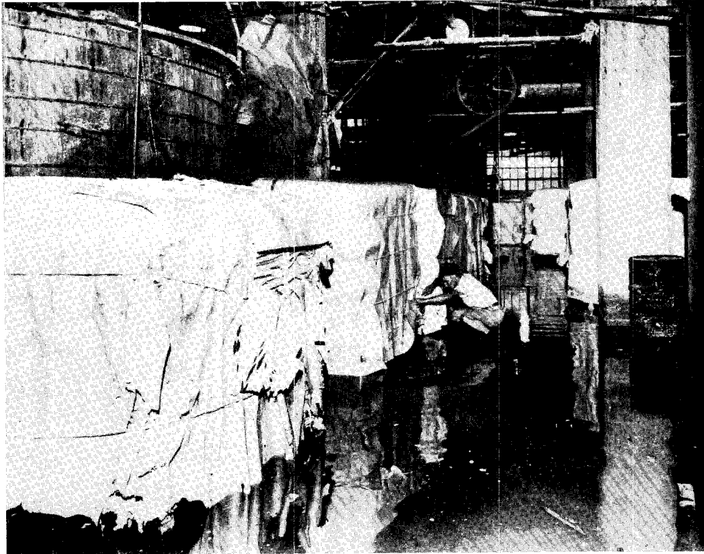
Figure 2.--AFTER THE MID-AUGUST 1940 FLOOD ON PIGEON RIVER Inside the plant of the Champion Paper and Fibre Company at Canton. The late August flood was about 3 feet higher than the flood line shown in the picture. (Photo courtesy "Asheville Citizen-Times")
