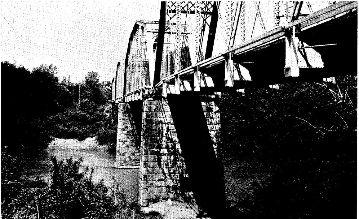
FIGURE 2. CAPE FEAR RIVER BRIDGES
