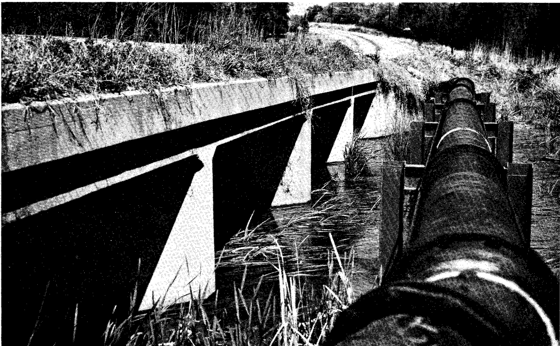
FIGURE 7. CROSS CREEK BRIDGES
