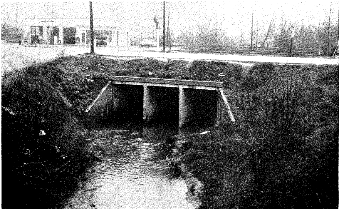
FIGURE 10. BLOUNTS CREEK BRIDGES
