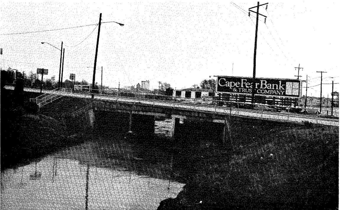
FIGURE 6. CROSS CREEK BRIDGES
