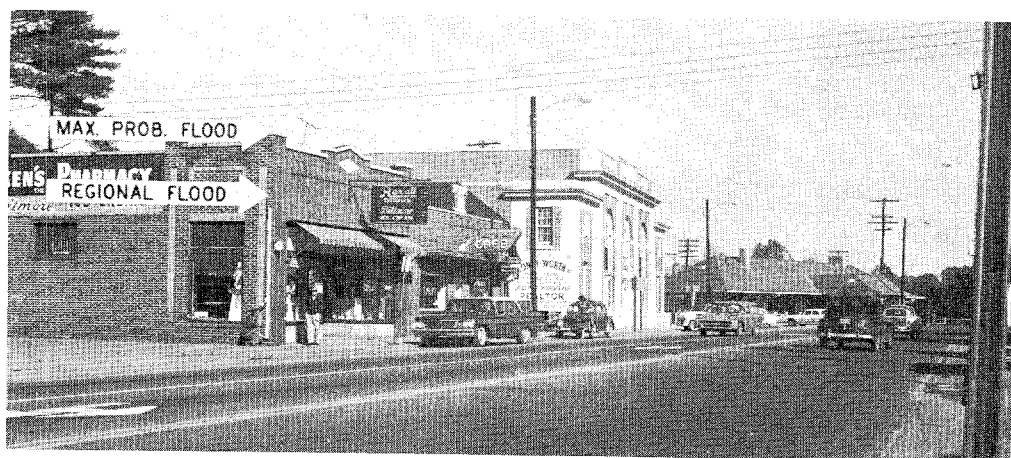
Figure 28. --OFFICE BUILDING, POST OFFICE, AND STORES IN BILTMORE
