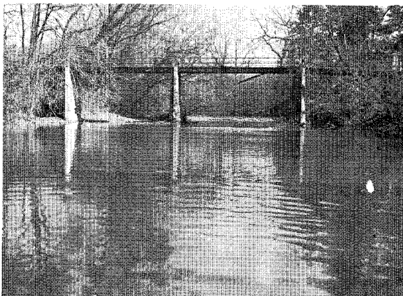
Cheeseborough Bridge, Mile 3.12, downstream side
