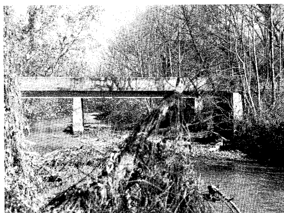
Azalea Bridge, Mile 6.97, downstream side
